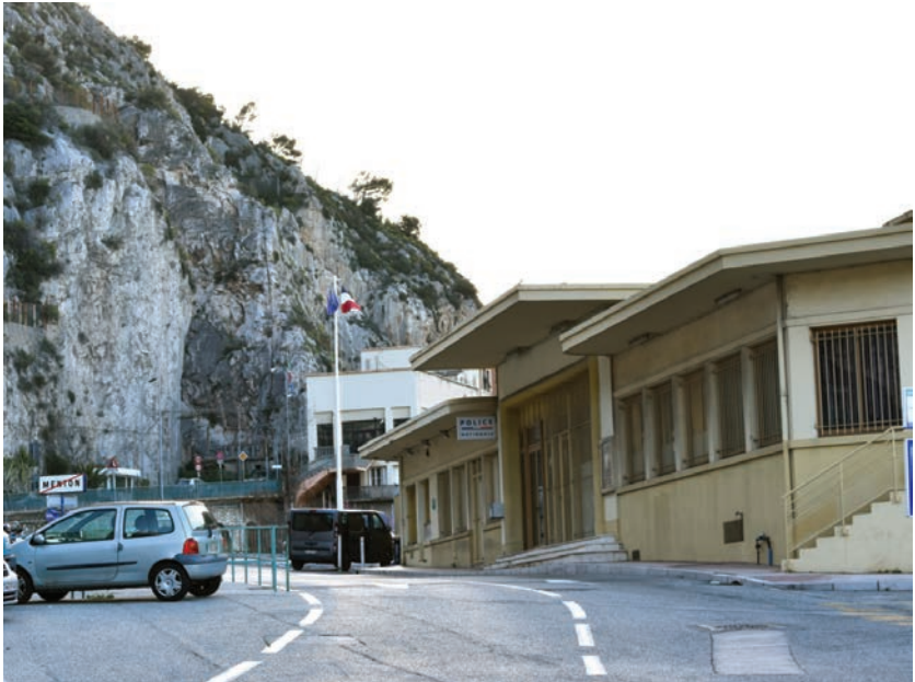
PAF (POLICE AUX FRONTIÈRES) OFFICES AT THE MENTON BORDER, WHERE MIGRANTS CAUGHT AT THE BORDER ARE DETAINED BEFORE BEING SENT BACK TO ITALY.
